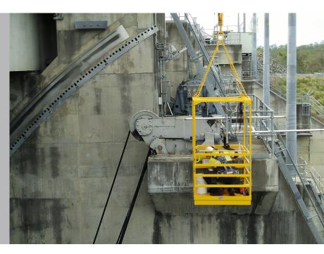
The project involved engineering assessment of the mechanical, hydraulic and electrical systems for the ten winches, including back-up hydraulic systems.
