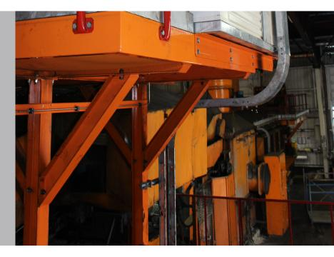
This required Practical Engineering to redesign Bandag's oil reticulation and dosing systems. We designed a heat traced and lagged ring main system to allow recirculation of heated process oils, as well as batch weigh vessels to allow batch weighing and delivery to their mix system.
